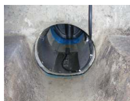
Installation of sensor in tube
